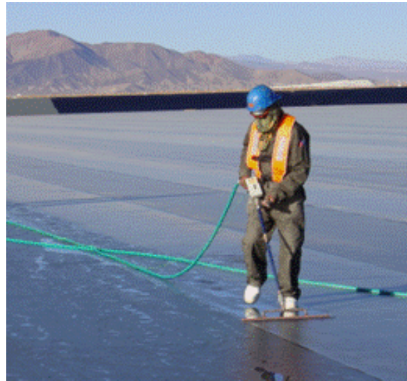
Figure 4. Leak location survey using the water puddle technique
